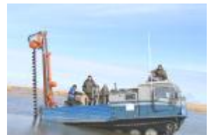
Drilling Module LITO-3
